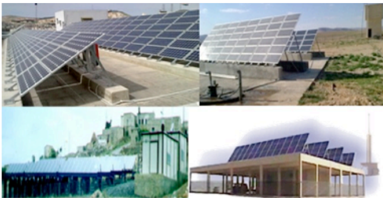
Figure 1: PV Systems installed in Syria.
