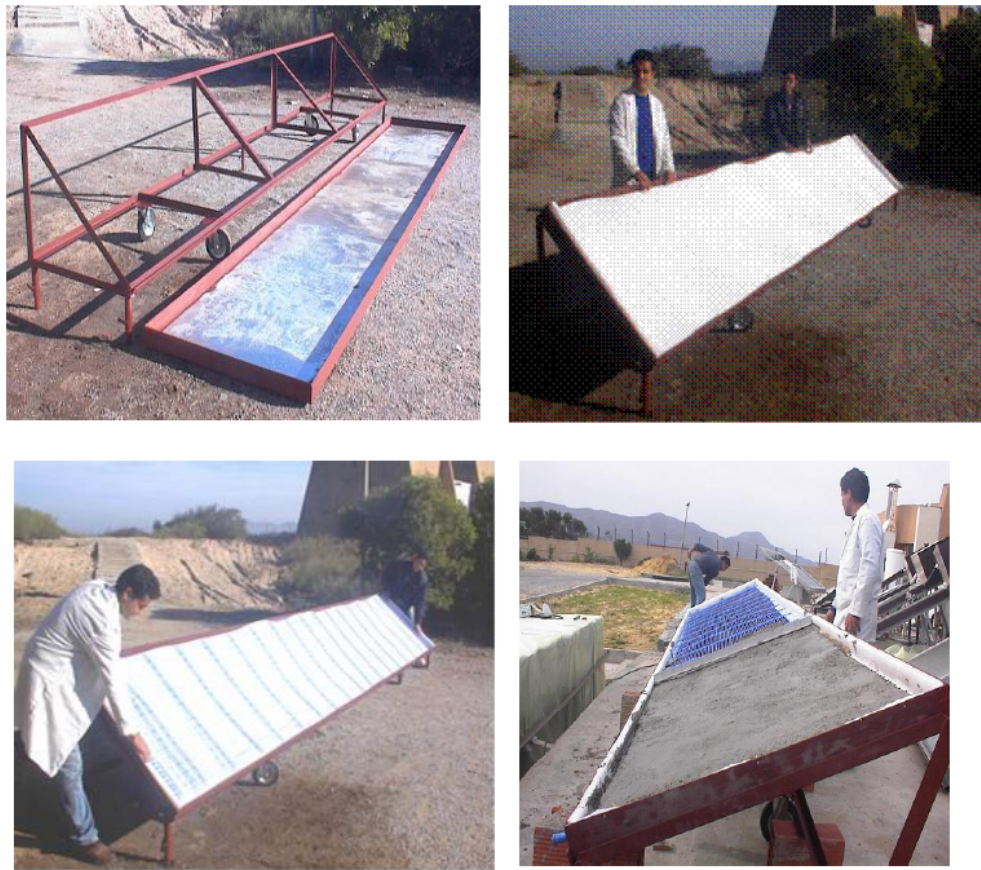
Figure 5: Different stages of the solar storage collector construction.
