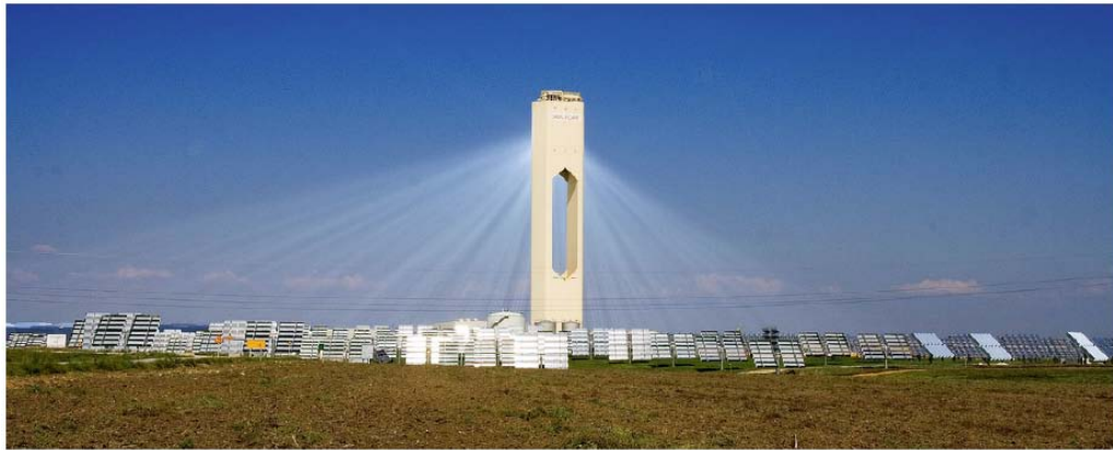
Figure 3: Solucar PS10, the first solar thermal power plant based on a tower in the world that commercially generates electricity.
