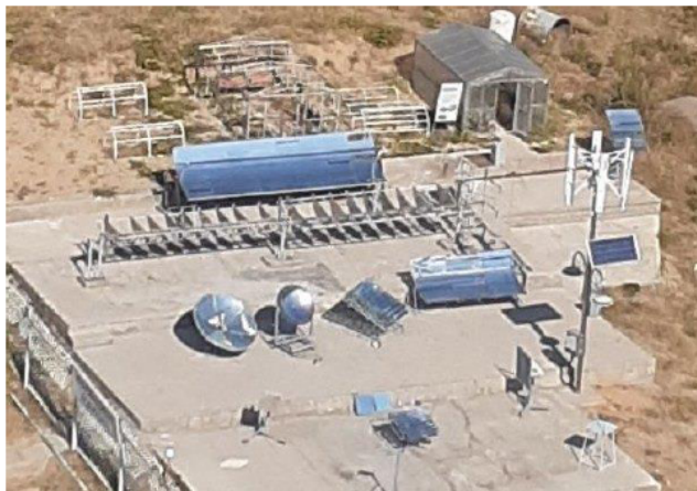
Figure 1: Innovative polygon with small solar concentrators, hybrid: wind-solar combined installation.
